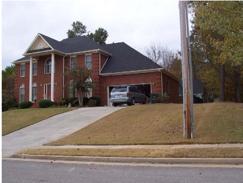
Photo 1: An upslope house with no connected roof drainage, sidewalk example, and telephone pole.
